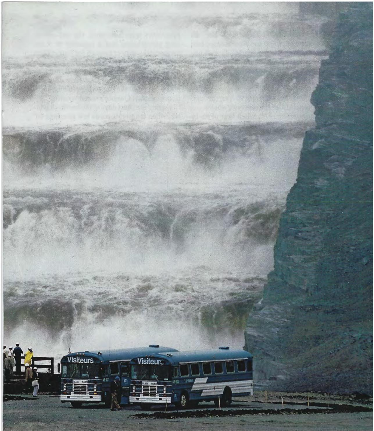
**T**AMED AND HARNESSSED, the rivers of northern Quebec are being put to work in the most monumental hydro-power project ever undertaken in North America. As visitors from Montreal look on, spillover from a giant new reservoir cascades down a man-made canyon at LG 2, largest of three colossal dams along La
